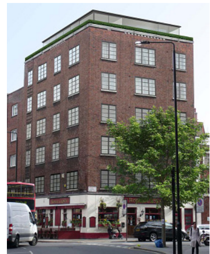
Gwynn House, Chelsea -Refurbishment of residential apartments and new penthouse
